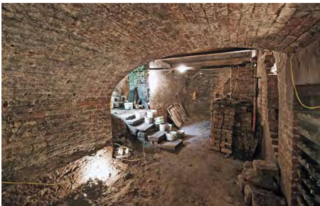
Elliptical Arch section of the Wine Bins under Williamson's House site
